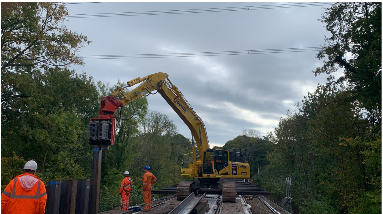
Figure 1: The Komatsu PC490 with Movax SG75V side grip attachment
